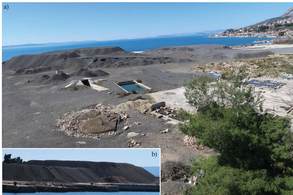
Slika 5. Pogled s kopna (a) i s mora (b) na ostatke nekadašnje tvornice karbida i ferolegura Dalmacija – Dugi Rat / Figure 5. View from land (a) and from the sea (b) of the remains of the former Dalmacija – Dugi Rat Carbide and Ferroalloy Factory
